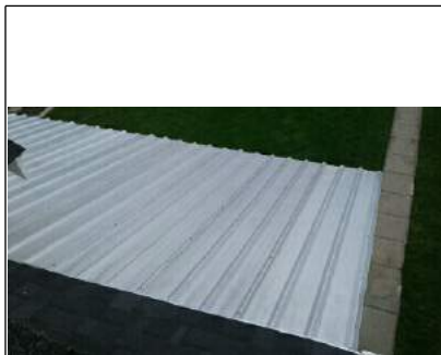
Example of patio roof covering
