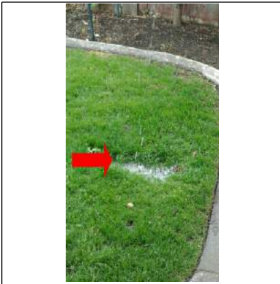
Example of needed downspout
